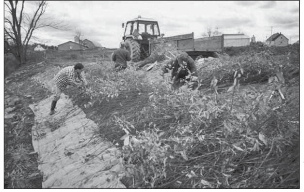
Photo 16: Installation de matelas de branches
